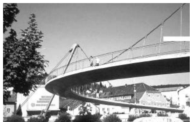
Figure 7 Kelheim Foot Bridge
